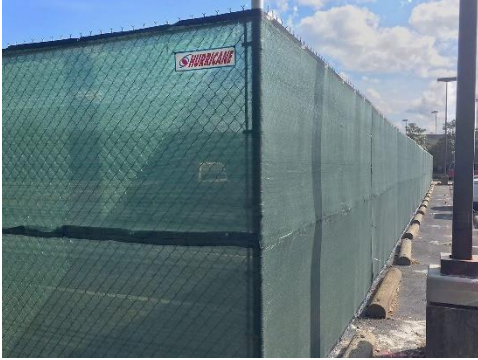
Example of a temporary construction fence
